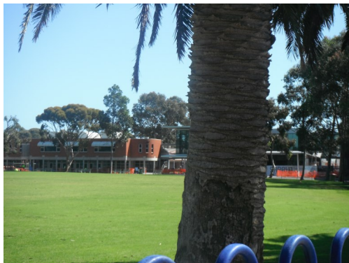
Behind the red brick building was another similar building which was the dining room.
