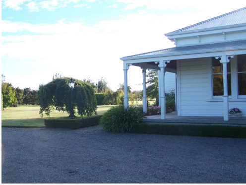
Front view of where the addition is to be -
